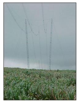
Cross-rope SuspensionTower Design
